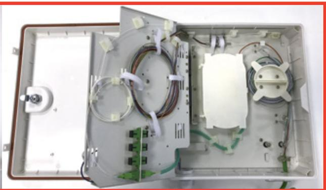
This box is used as a connection to the network (power cable) and / or a termination point with OLOs. The distribution cable is also installed with loop mode. The box can be used as a reference point, division or distribution of the fiber. It is perfect for networks in FTTH networks. It can be used inside.
