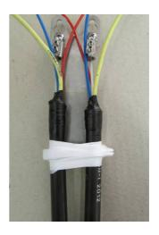
4.2.2.8 Make a coil of the continuous tubes of the cable and pass them through the heat-shrinking sleeve in the kit OF0049, taking care to not damage the internal part interna of the sleeve and the adhesive
