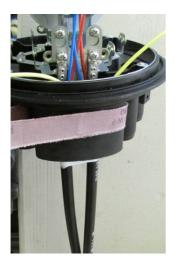
4.2.2.11 Deeply clean with the small towel and abrade the surface of the cables with the abrasive cable
