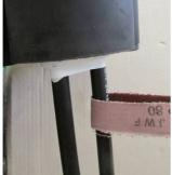
4.2.2.12 Put in position the heat-shrinking sleeve as far as the base of the splice closure and mark the cable as in the picture
