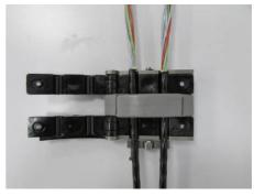
4.3.2.6 Close both the plastic jaws tightening the TC screws and reposition the upper and lower steel plates
