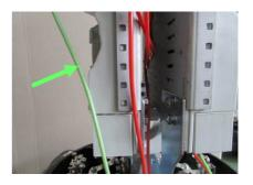
5.2.2.2 Wrap the continuous tubes of the cable in a skein and fix them in the central area between the 2 frame and fix it with plastic cable tie.
