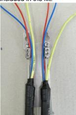
4.2.2.6 If the cable diameter is > 8mm fix the cables to the bracket using the metal screw clamps of the kit, otherwise (if D < 8mm) use the cable ties in plastic.
