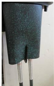
4.2.2.15 Heat-shrink the sleeve starting from the top part leaving it rest for about 2 minutes
