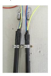
4.2.2.7 If the metal screw clamps are used, use the Teflon tape in the kit to cover the screw clamps themselves so that the sleeve is protected during the heat-shrinking
