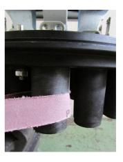
4.2.1.9 Put the heat-shrinking sleeve in position as far as the base of the splice closure and mark the cable as in picture.
