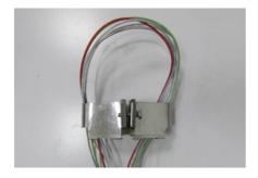
4.3.2.5 Open the pre-cut gasket and insert the two parts of the continuous cable into the kit body so that the cable routing is in line with the upper exit of the kit body.
