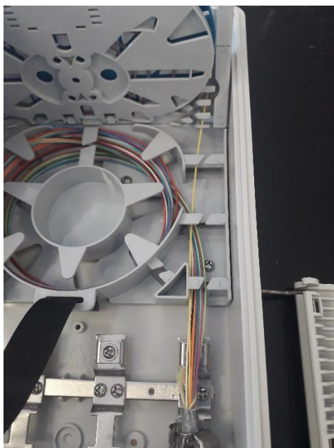
19. Move the 900um fiber to splice passing through all right retainers, going to splice trays.
