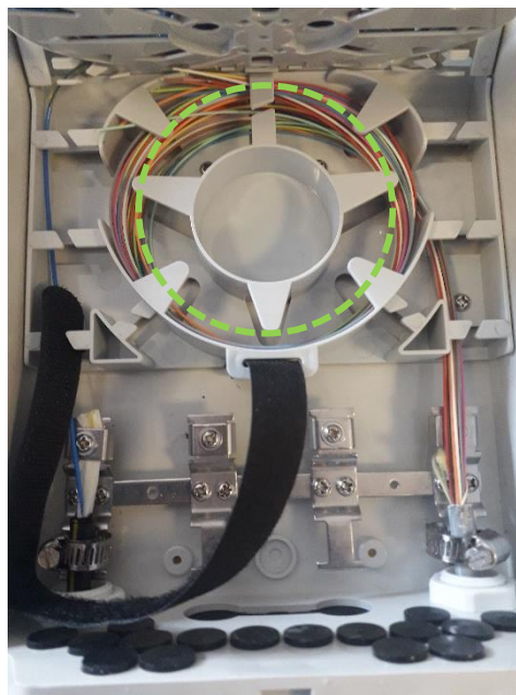
18. Store the unused fibers on the central cable manager.
