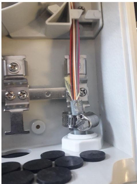
17. Fix the multifiber building cable on the right side.
