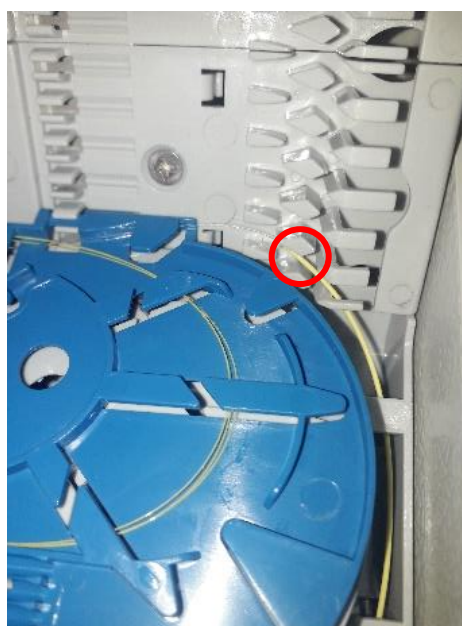
20. Strip the 900um jacket and come in splice tray holder.
